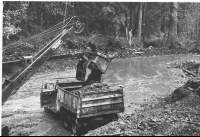
1960s: extracting gravel from Twelvemile Creek to use for road construction
