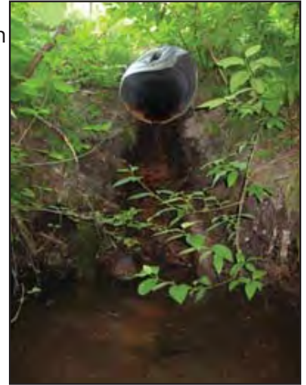
Cannery Road Culvert
